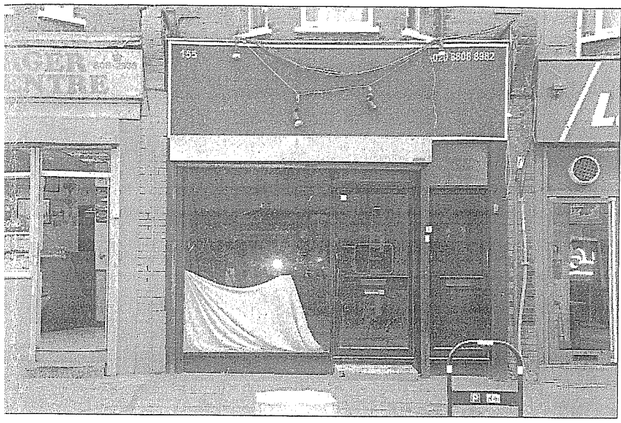
Front of Shop
